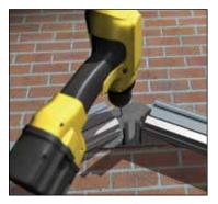
The ridge hanger/compression plate is attached to the host wall using two anchor bolts (not supplied).
