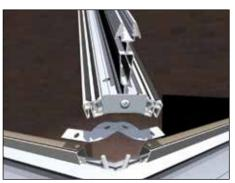
On Georgian / 90° corners, a butterfly cleat is laid over two captivated roofing bolts. Note: A butterfly cleat is not required on 3 or 5 facet fronts unless the eaves beam joins a box gutter at the facet joint.
