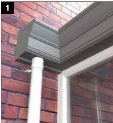
**1** Return Cornice and guttering along host wall.
