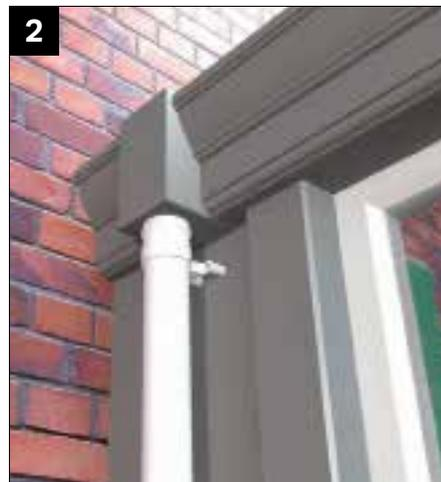
**2** Elephants Trunk outlet. If it is not possible to have full height columns i.e. on dwarf wall.
